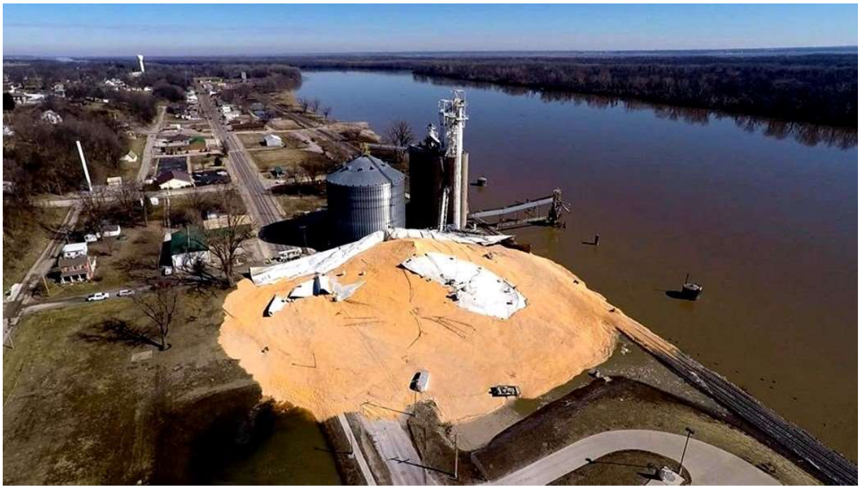
INVESTIGATION OF THE COLLAPSE OF A GRAIN BIN
